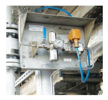
The oil & gas companies do have specific pneumatic circuitry for control panels and systems to operate pneumatic actuated utility- and process valves. With our compact modular system we easily build and comply with any specification and sizes.
